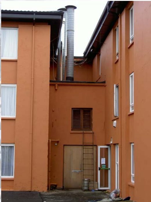
Figure Pre-installation image
