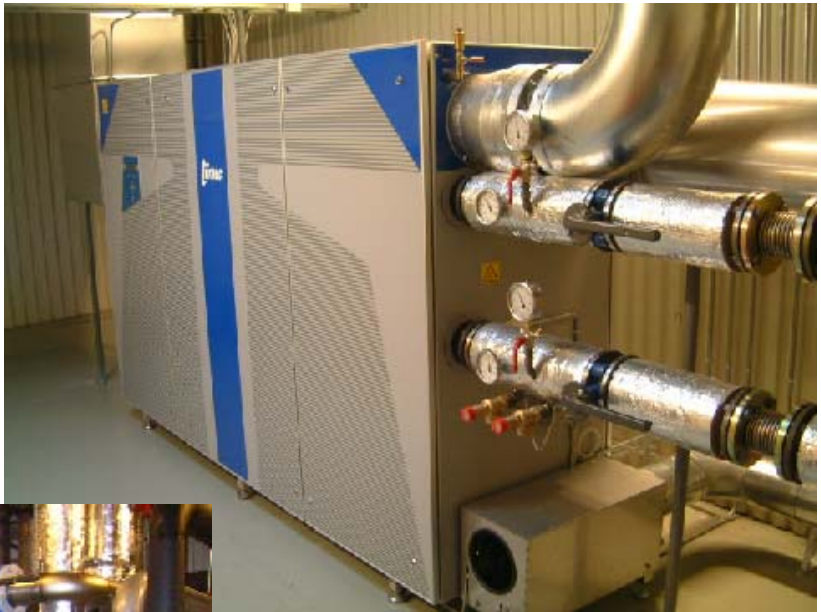
Turbec T100 at Statoil, Forus, Stavanger. Photo: Roar Stokholm, Statoil
