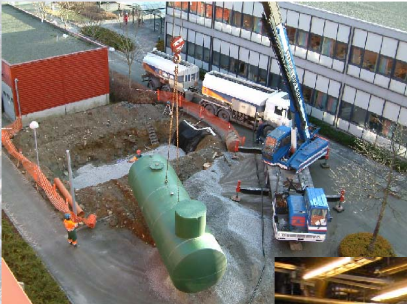
Installation of methanol fuel tank at Forus. Photo: Tor Berquist, Statoil
