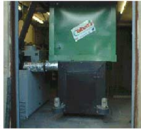
Figure 8 (l): Schematic of combustor & heat exchanger ®: picture of combustor connected to microturbine, with biomass silo on top
